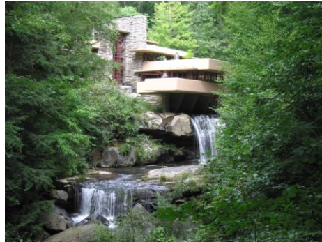
Gambar 2. Frank Lloyd Wright's Fallingwater Damaged from Flooding Sumber : www.archdaily.com (diakses 1 Desember 2019)
